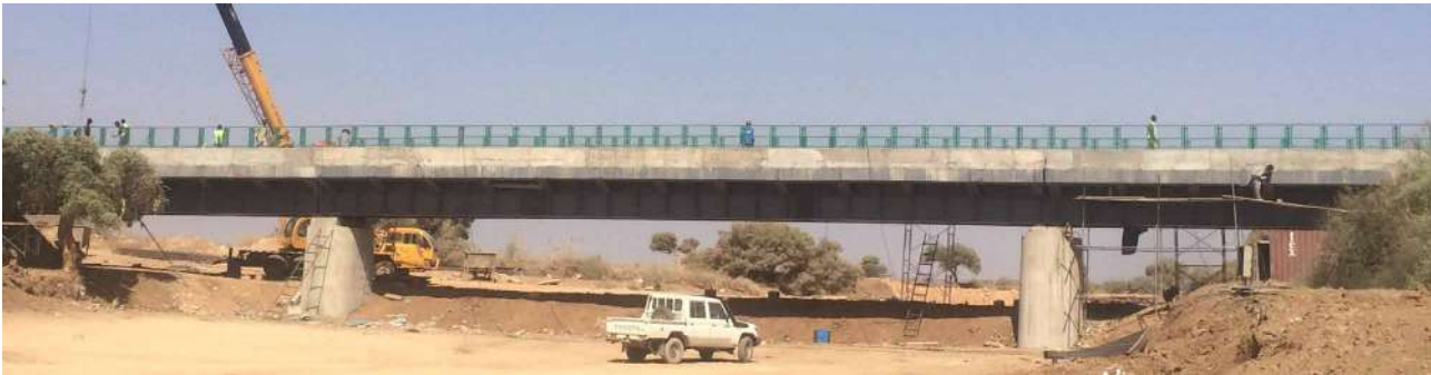
埃塞俄比亚DABOWEIN大桥 Ethiopia DABOWEIN Bridge 钢结吨位: 300余吨。 特点: H型钢梁简支梁三孔桥, 跨径为18.5+30.5+18.5米。 Steel structure tons: 300 tons Features: H type steel beam bridge with 3 openings, span is 18.5m+30.5m+18.5m
